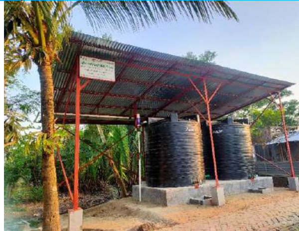
3. Fully construction of Rainwater harvesting system
