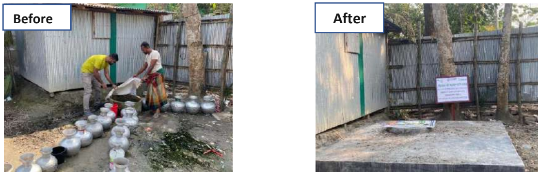
Figure 10: Repair and reconstruction of the municipality's water collection point
