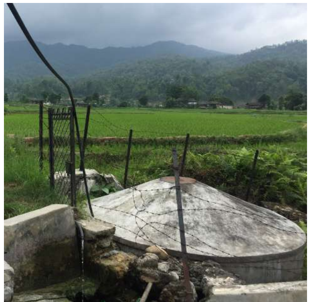
RVT tank impacted by Flash flood at Hilepani community, Sindhuli.JPG
