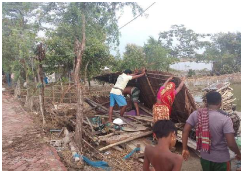
Figure 4: Many Locals of Dakshin Bedkasi areas have lost their house, affecting their life and livelihood after Cyclone Yaas hit the area, photo taken on 7th June, 2021. Courtesy Sufiya Khatun
