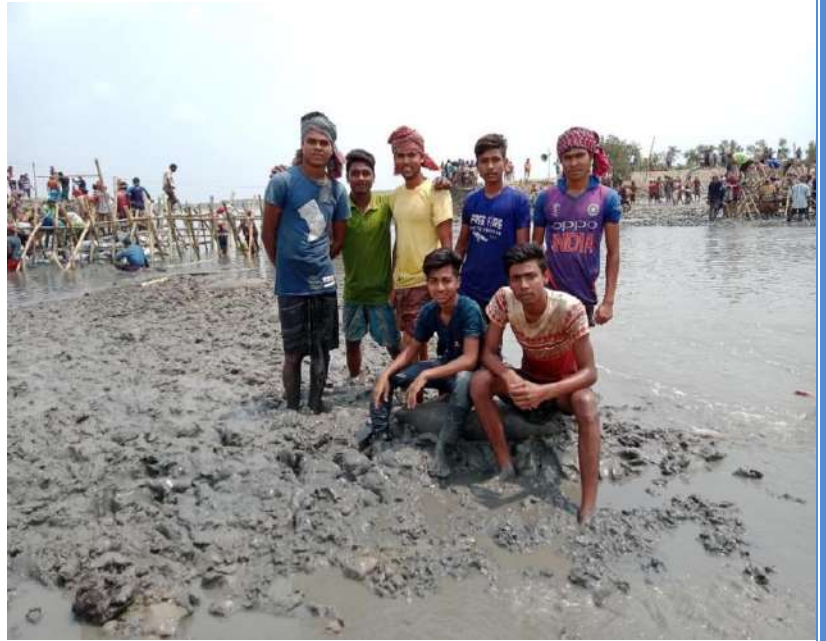
Figure 7: After Cyclone Yaas, local youths self-organized to repair the embankment and resettled their home with their own initiative in the coastal region. Courtesy Vaskar Mondol
