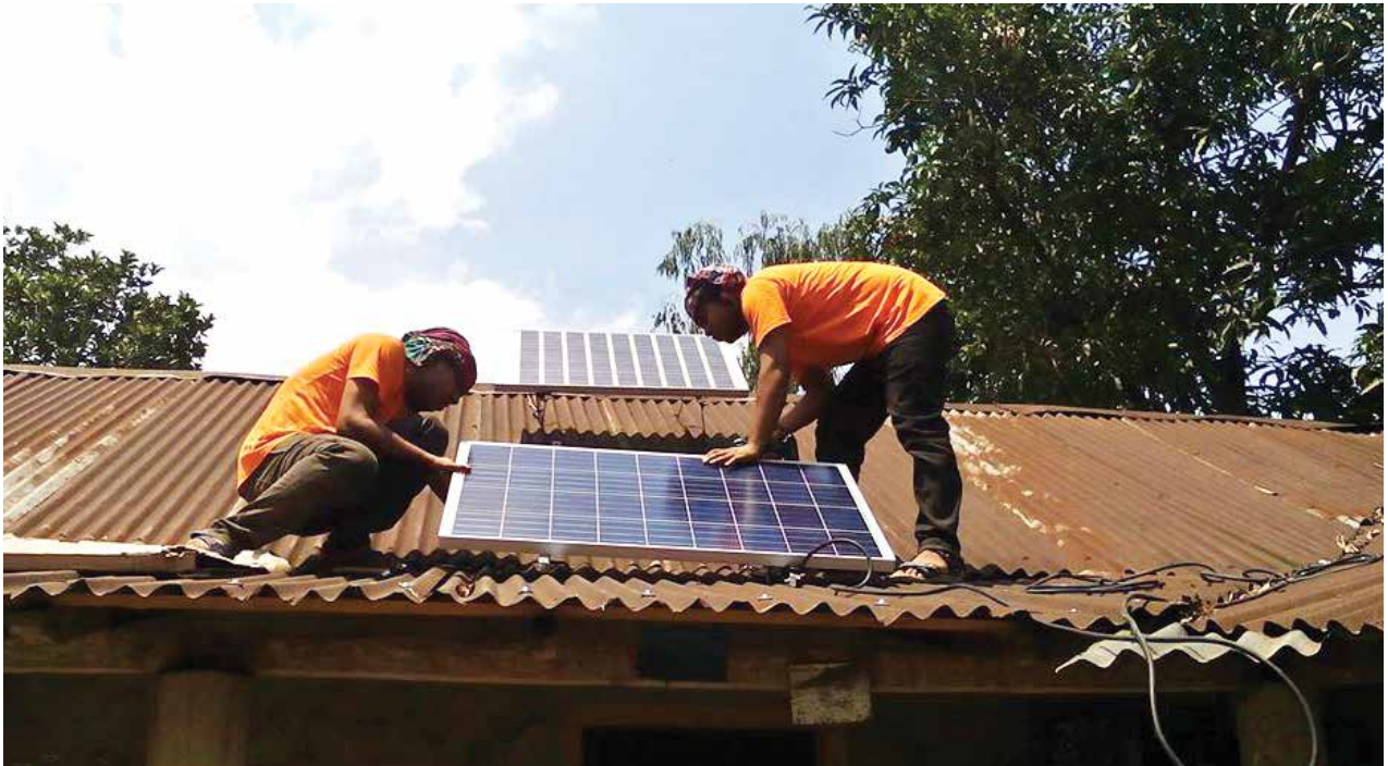
SOLshare technicians fitting solar panels
